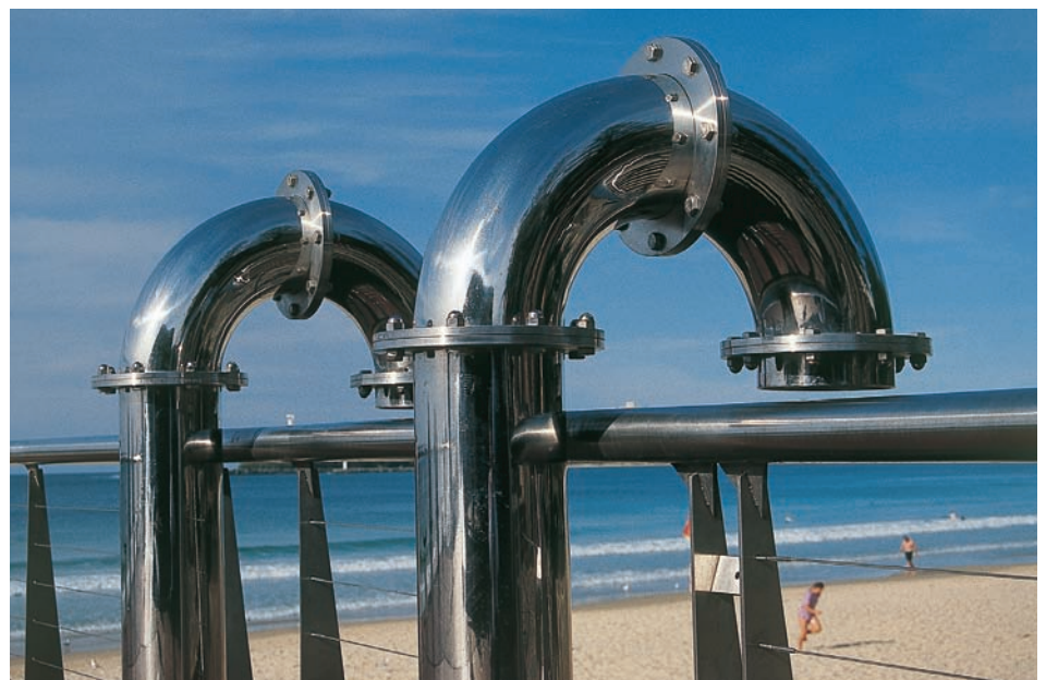
A successful stainless steel coastal application, with no tea staining.
